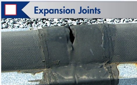
Check for signs of excessive movement, leaks, or deterioration.
