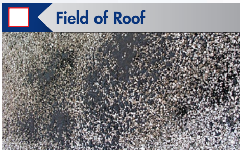
Redistribute ballast; note damage/deficiencies; inspect coating.
