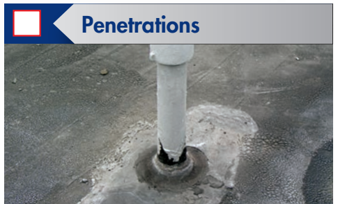
Fill all pitch pans; inspect pipe boots.
